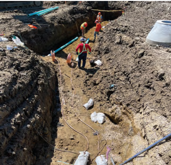
Crews installing water and sewer lot services.
