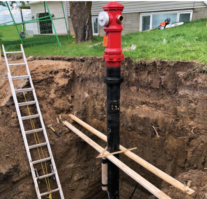
Installation of a fire hydrant.
