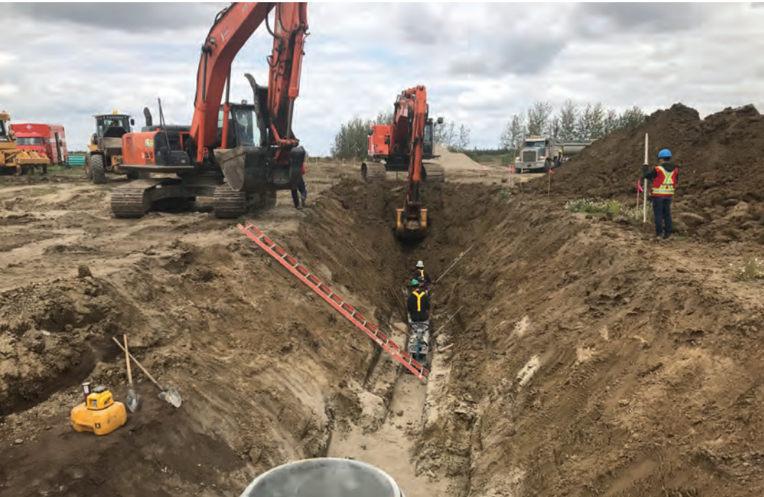
Crews installing sanitary sewer main and manhole.
